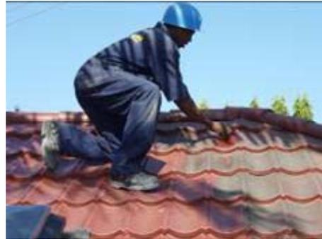
Method: Work from the apex (top of the roof) down. Use only recommended Solution. Use a NYLON scrubbing brush dipped in the solution to scrub free dirt/algae growth. After 1 hour scrub tiles using clean water.
